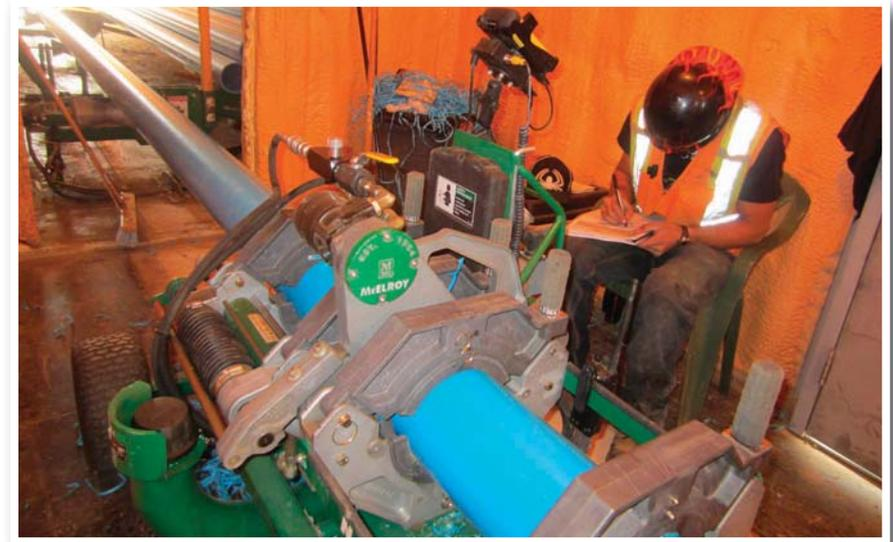
*Shipping container shelter configuration used for fusing in winter conditions.*
